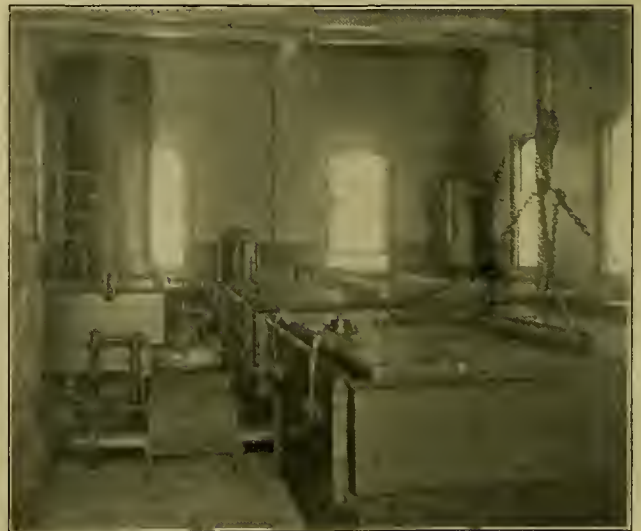
Fig. 6.—Condenser, Washer and Purifiers.
